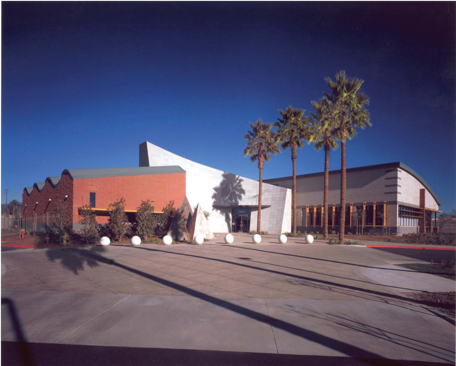
The Cucamonga Valley Water District Main Office at 10440 Ashford Street, Rancho Cucamonga, California
